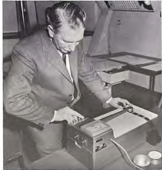
A densitometer being used for checking film gradation and quality. Keeping a watchful eye on things is Mr. Bill Griffiths ( head photographer ).
