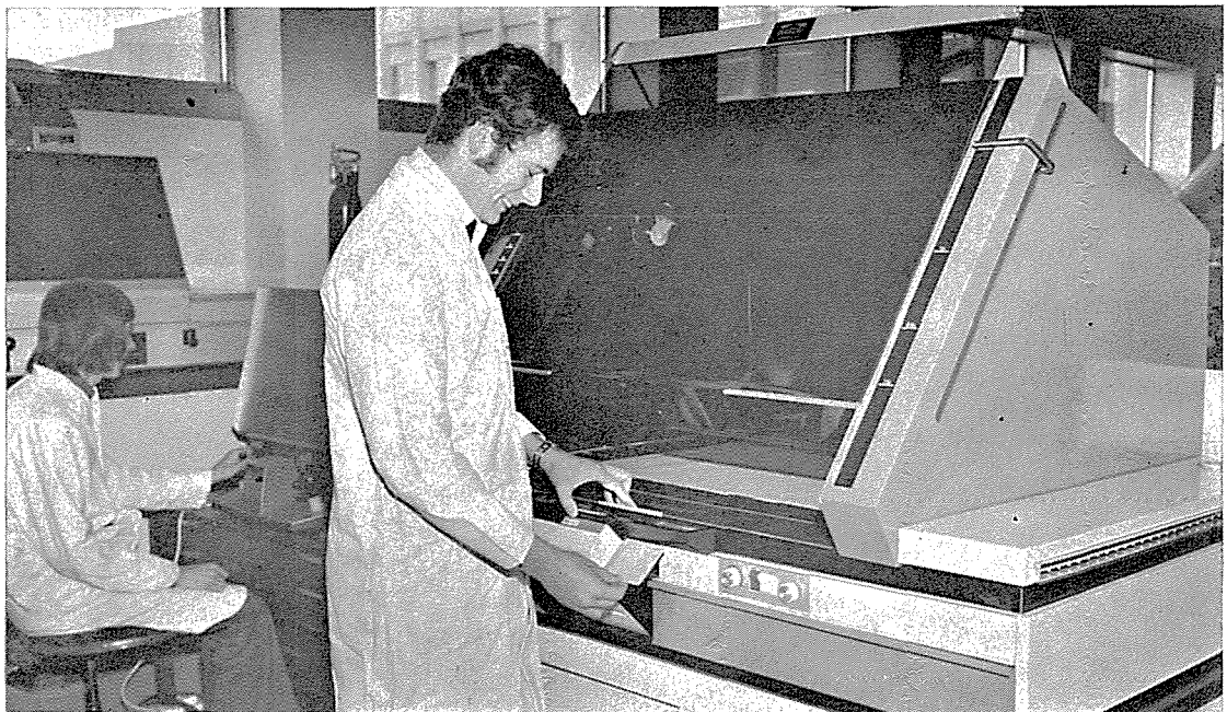
Mrs. Margaret Edwards, above , producing duplicate working aperture cards from an original 35 m.m. silver image film, which is kept as the master copy. Mr. Adrian Chesworth, below, left , extracting information with the aid of a viewer, while Mr. Howard Pearson inserts an aperture card into an electrostatic printer which in about ten seconds, produces a full-scale reproduction on paper.
