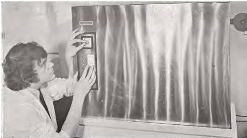
Exposed film being fed from a cassette through the fully automatic processor. This unit develops 100 feet of 35 m.m. film (600 exposures) in 25 minutes. The operator in our picture is Mr. Mike Hall ( staff photographer ).
